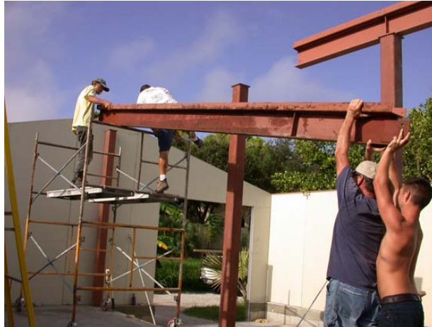
Home Front Homes – Ridge Beam Installation
