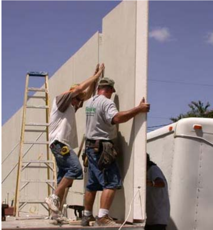
CSIPs being erected during a residential construction.
